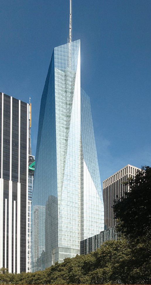
Waste heat from a gas turbine will be used to heat and cool the Bank of America Tower.
